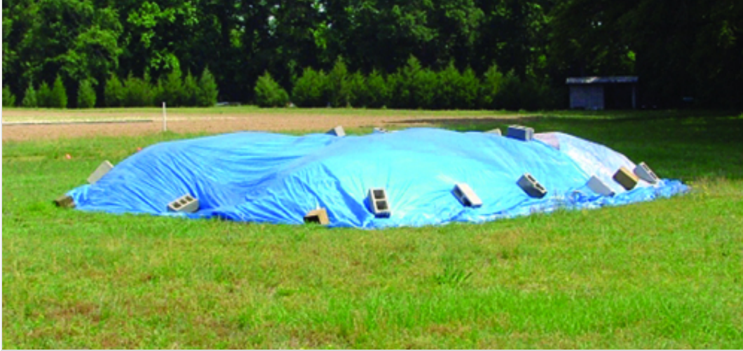
Fig. 1. Use of a tarp to cover stockpile. Photo credit: Virginia Cooperative Extension.
